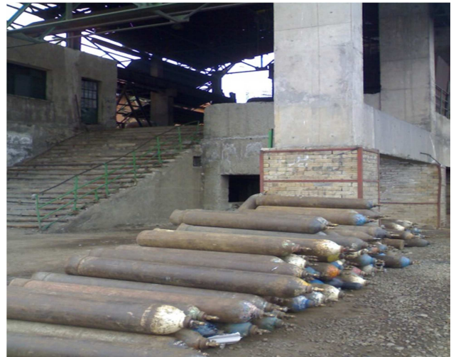
Figure 2. Oxygen cylinders position before the intervention
