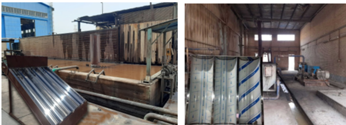
Figure 2: Solar hot water production system of hot water production system with weather conditions of Ahvaz..
